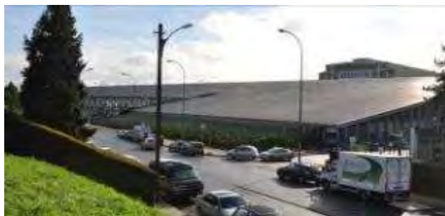
Figure 84 : parking et passerelle (APEB, 2011)
